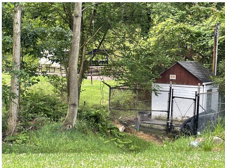
Collins Road pump station
